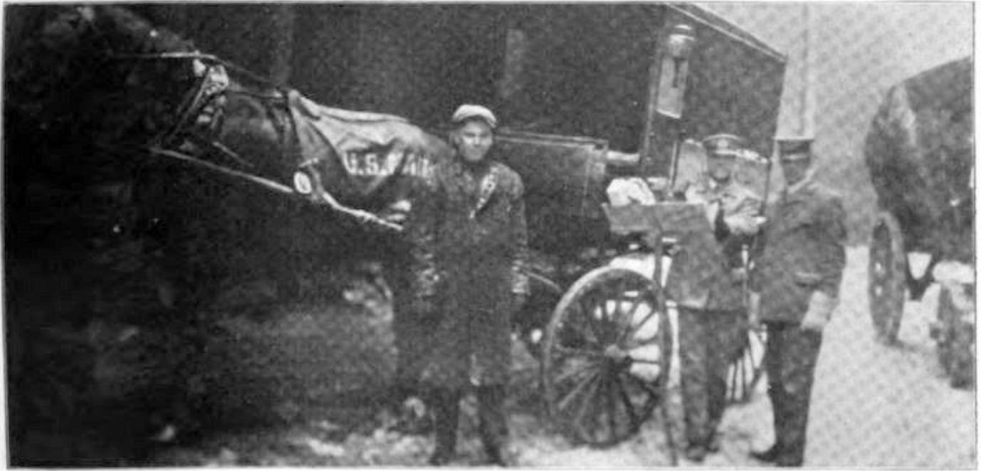
U. S. Postal Clerks Pressed Into Service as Hod Carriers Delivering Parcel Post Brick to Exposition.
